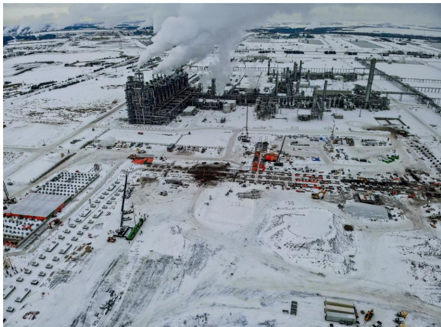
Existing Ethylene Cracker & concrete pilings for the 2 nd Ethylene Cracker
